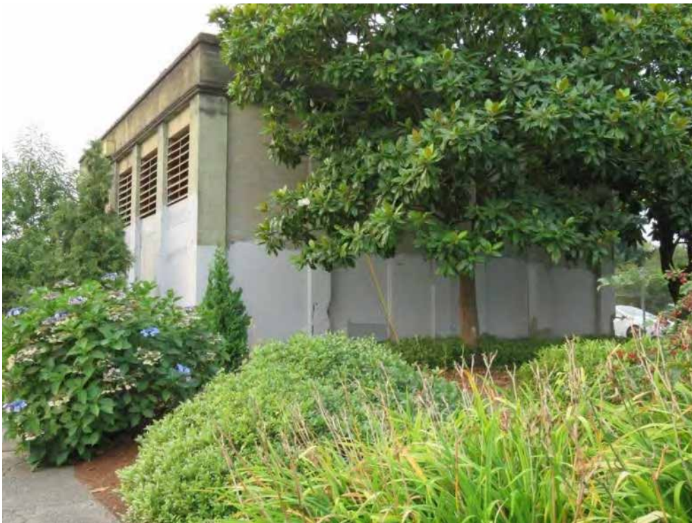
Photo 7 of 13. WA_PierceCounty_AdamsSt.Substation_0007. Adams St. Substation, oblique, view southwest.
