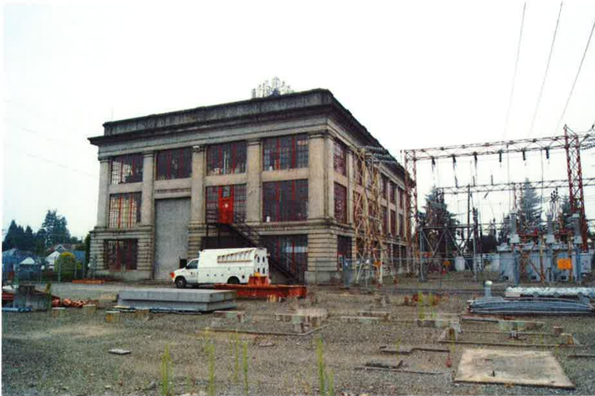
Photo 7 of 17. WA_PierceCounty_CushmanSubstation_0007. Northeast oblique of Cushman Substation, viewing southwest.
