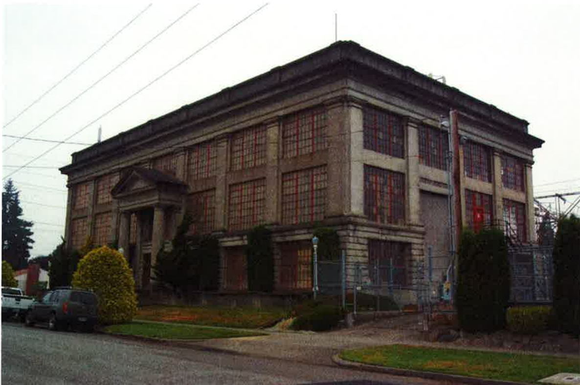
Photo 1 of 17. WA_PierceCounty_CushmanSubstation_0001. Cushman Substation, southeast oblique, viewing northwest.
