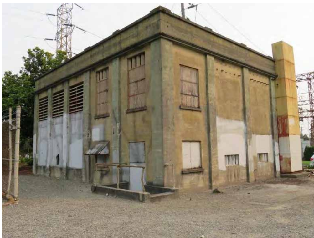
Photo 4 of 13. WA_PierceCounty_AdamsSt.Substation_0004. Adams St. Substation, oblique, view northeast.
