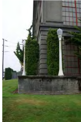
Detail of light poles
