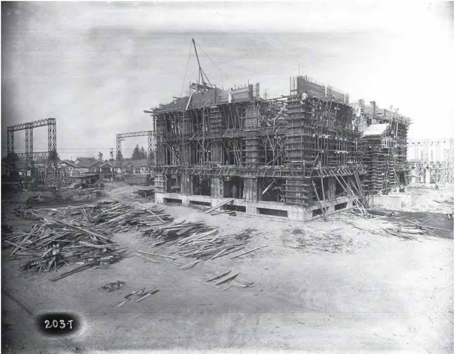
Figure 3 Cushman Substation under construction, board formed construction, August 3, 1925, Image courtesy of Tacoma Power
