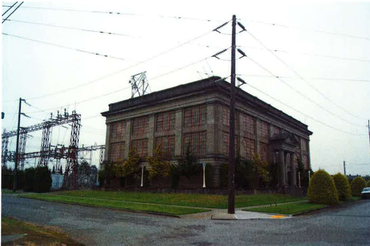
Photo 3 of 17. WA_PierceCounty_CushmanSubstation_0003. Southwest oblique of Cushman Substation, viewing northeast.
