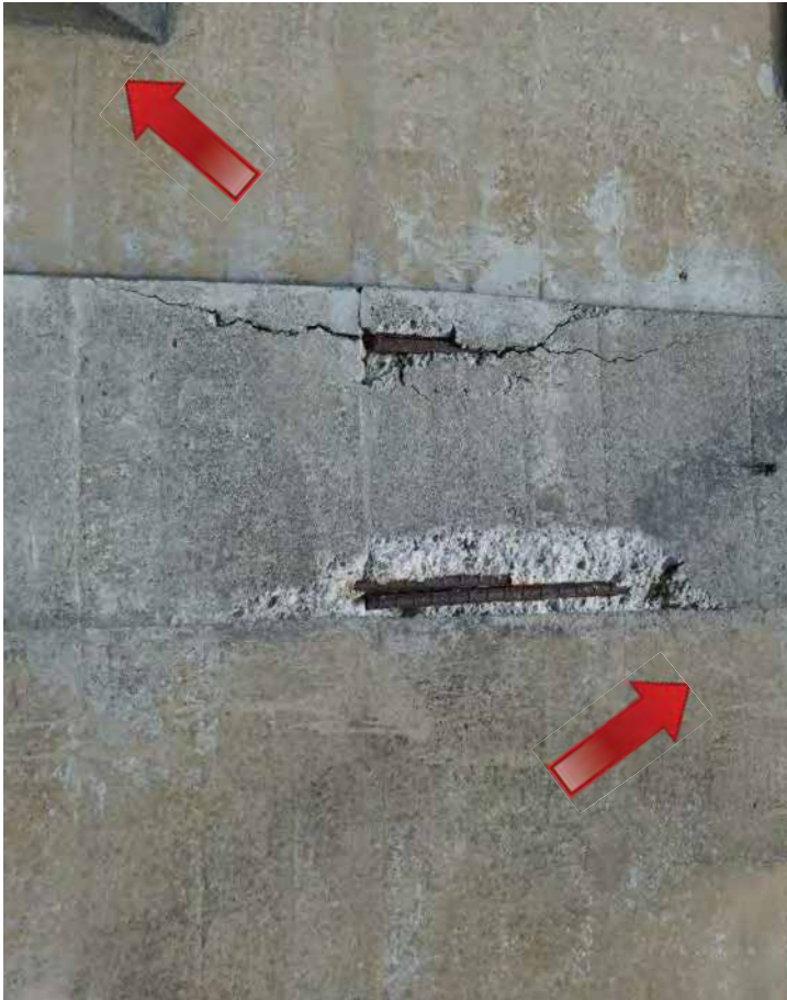
Discoloration of the yellow pigment is visible on all elevations on the building. Image by Richaven Architecture and Preservation. 220620 CoT CAS EL-W P1000681.JPG
