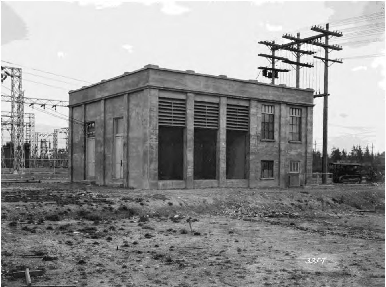
Figure 3. Adams St. Substation, nearing completion, view southeast, 1925. Courtesy of Tacoma Power.
