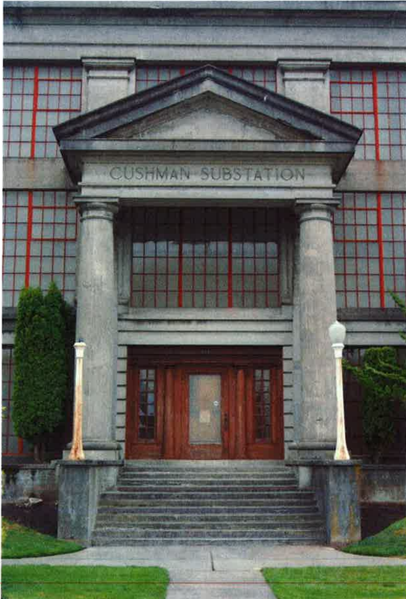
Photo 2 of 17. WA_PierceCounty_CushmanSubstation_0002. View of the temple front entrance on the façade (south face) of Cushman Substation.
