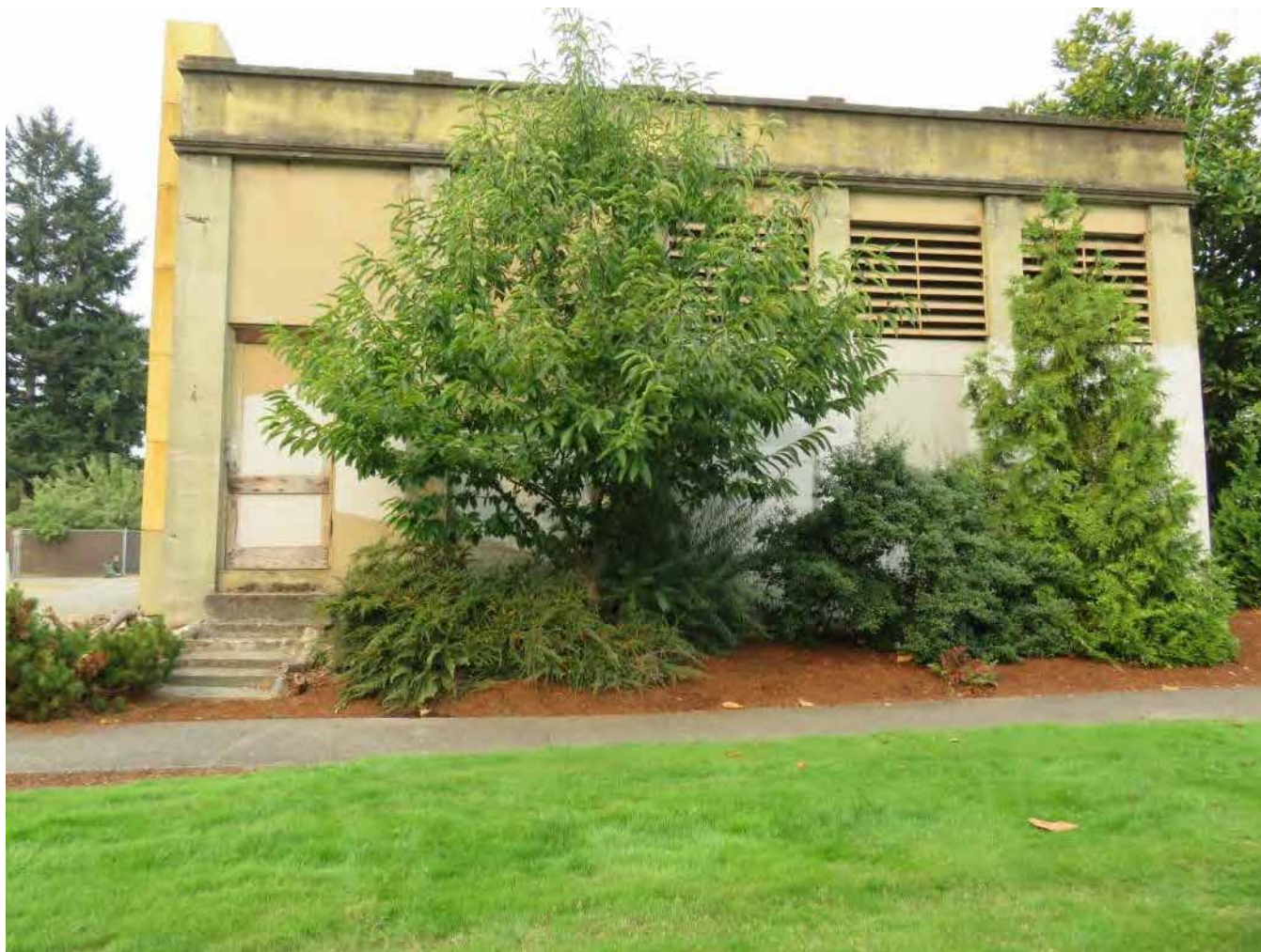
Photo 1 of 13. WA_PierceCounty_AdamsSt.Substation_0001. Adams St. Substation, primary façade, view west.
