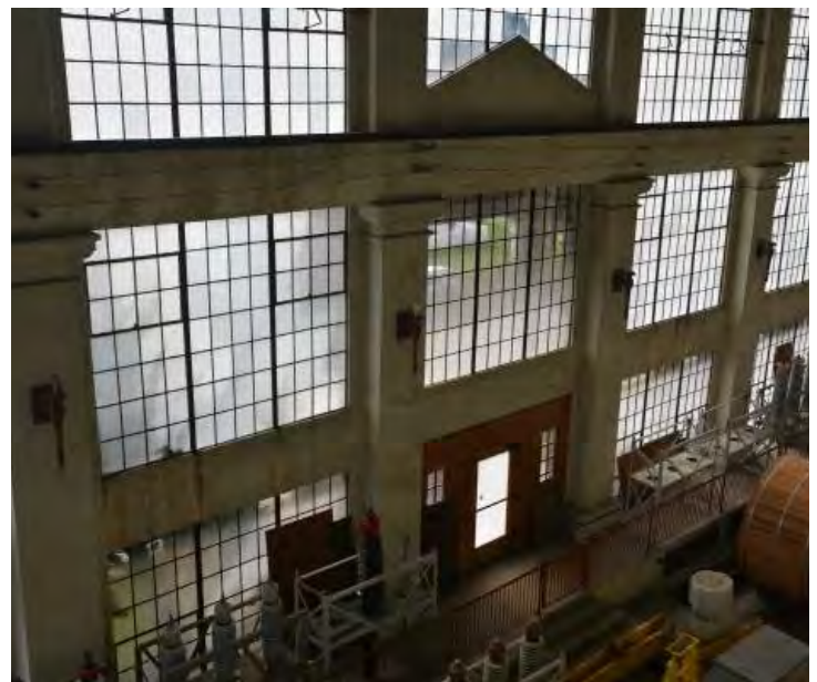
Glass globes are missing on the light fixtures above the main entrance. Image by Otak. 200224 CoT CAS EL-INT DSC_0999.JPG
