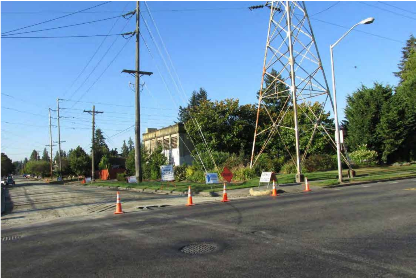
Figure 22 Adams Street Substation and Tower 1, view southwest
