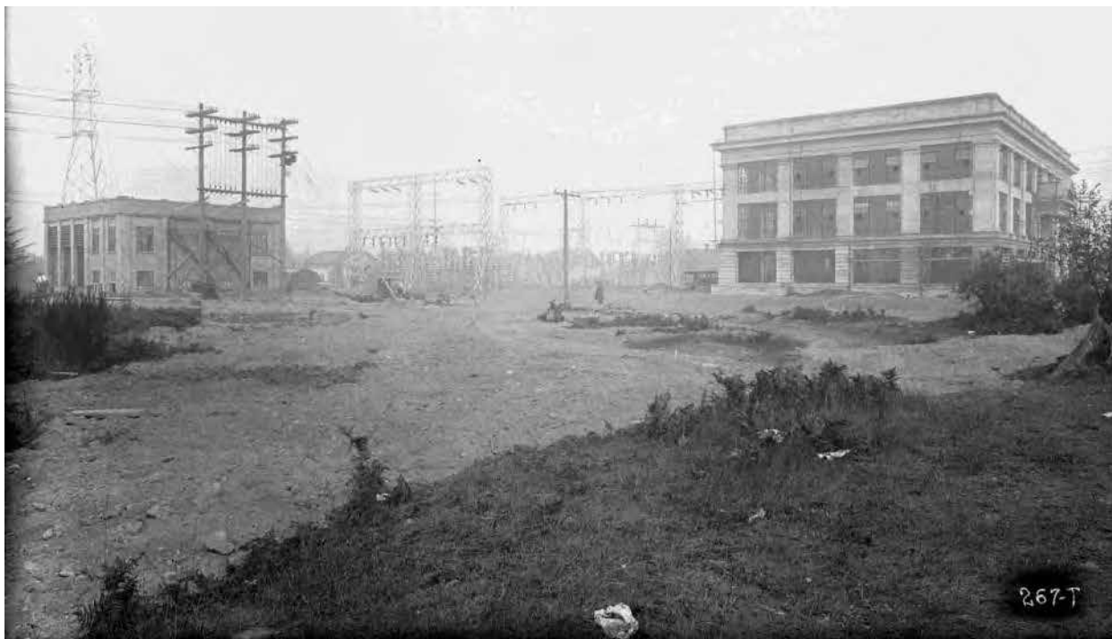
Figure 6. Adams St. Substation, shown beside Cushman Substation, view northeast, 1925. Courtesy of Tacoma Power.
