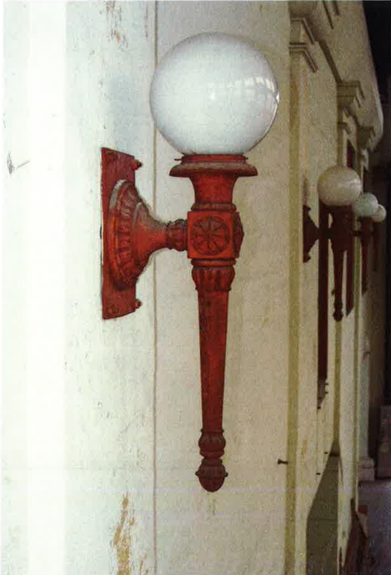
Photo 10 of 17. WA_PierceCounty_CushmanSubstation_0010. Detail of decorative light fixture at Cushman Substation.
