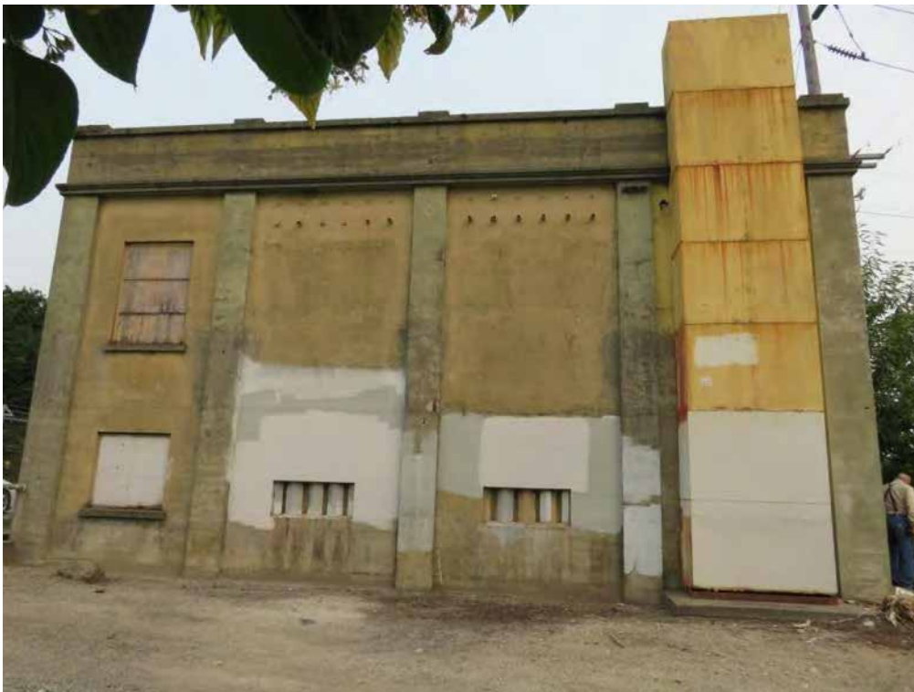
Photo 3 of 13. WA_PierceCounty_AdamsSt.Substation_0003. Adams St. Substation, south elevation, view north.
