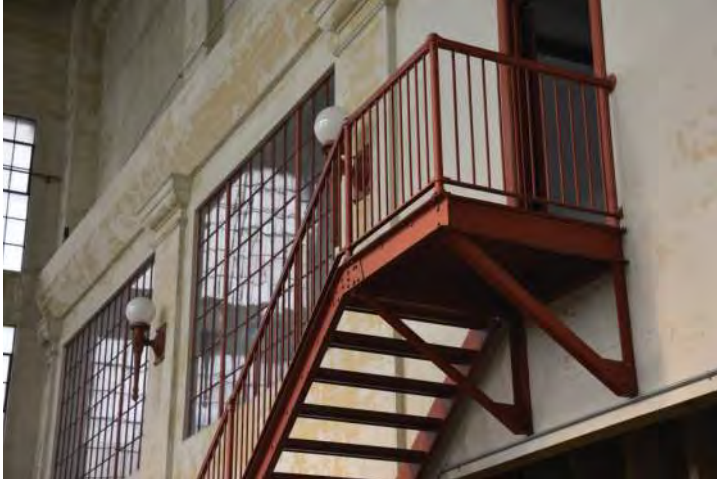
The stairwell railings are in fair condition. No corrosion was observed. Image by Otak. 200224 CoT CAS INT DSC_0977.JPG
