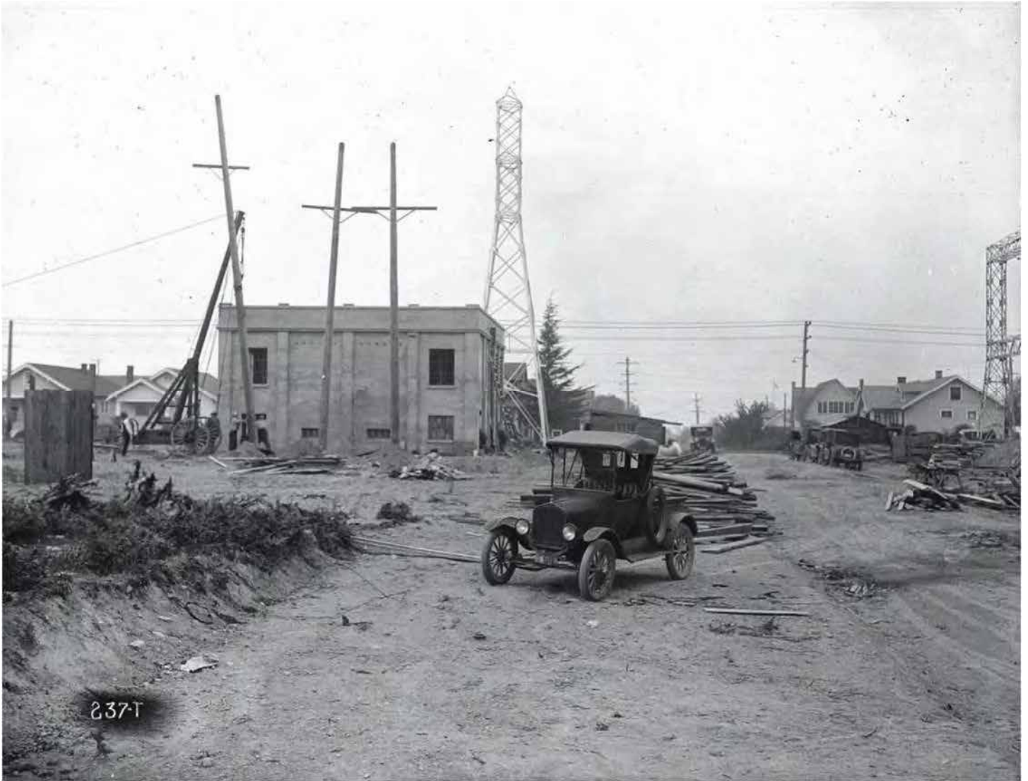
Figure 5 Adams Street view North, September 8, 1925, Image courtesy of Tacoma Power
