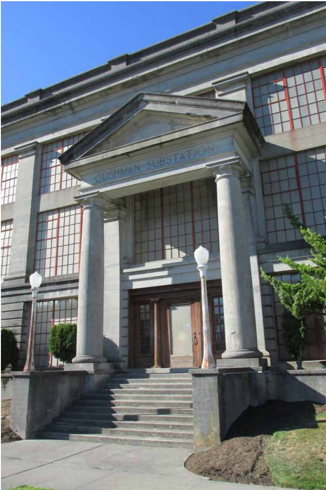
Figure 16 Cushman Substation, main entry onto 19th Street
