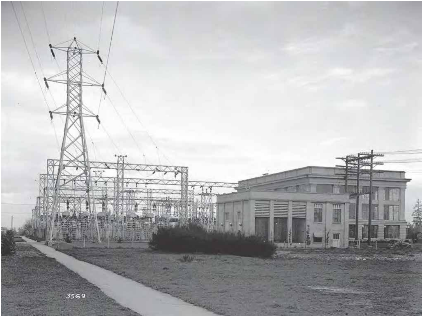
Figure 12 Cushman complex, View east April 13, 1937, Image courtesy of Tacoma Power
