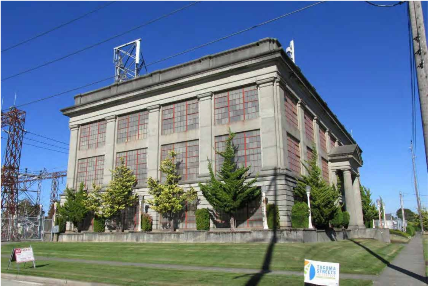
Figure 18 Cushman Substation, view northeast
